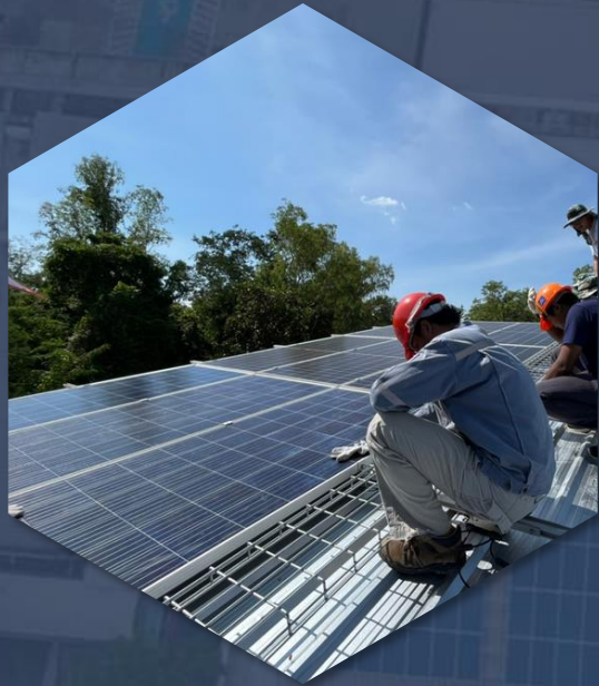
Walkway & fitting support
